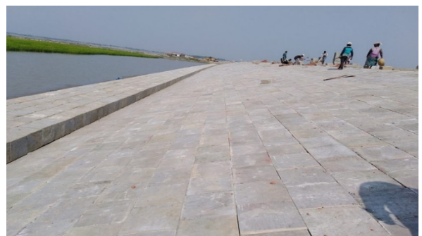
Figure 3-10: Completed Slope Protection Works in Polder-32
