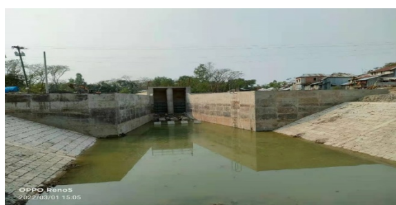
Figure 3-26: Slope protection work for km 32+015-34+300 in Polder-39/2C
