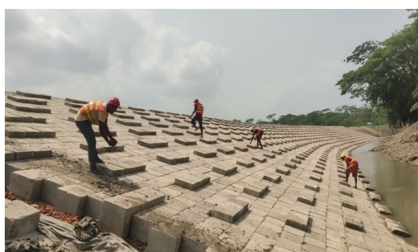
Figure 3-26: Slope protection work for km 32+015-34+300 in Polder-39/2C
