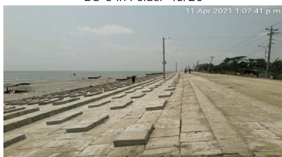
Figure 3-30: Slope Protection work from KM 30+800 to Km 31+450 in Polder-48
